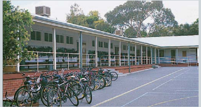
Six units installed at Coolbinia Primary School, Perth Western Australia.
